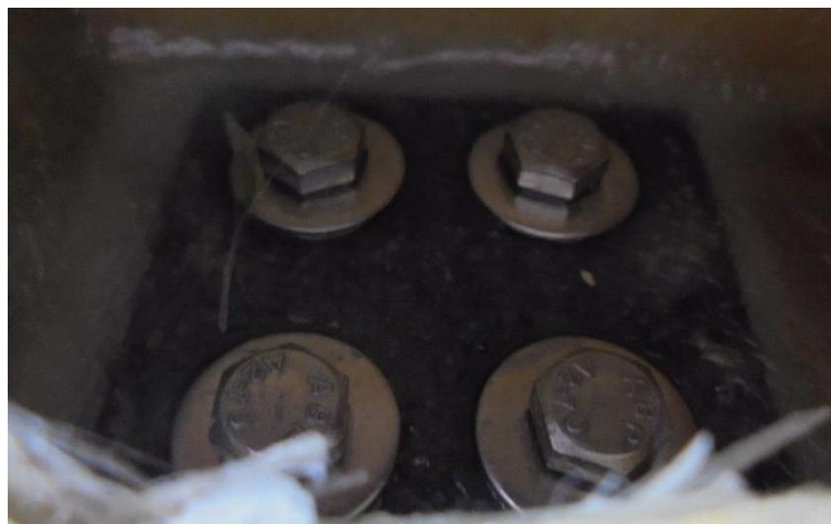
Figure 5: Bolts and washers installed
