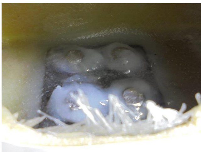
Figure 6: Thickened resin around bolt heads and washers with covering layers of glass fabric
