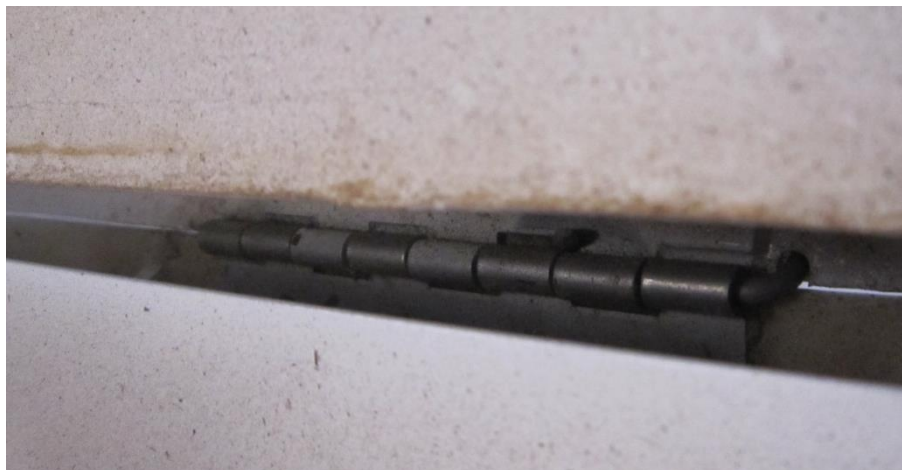
Figure 25 - Aileron hinge from above
