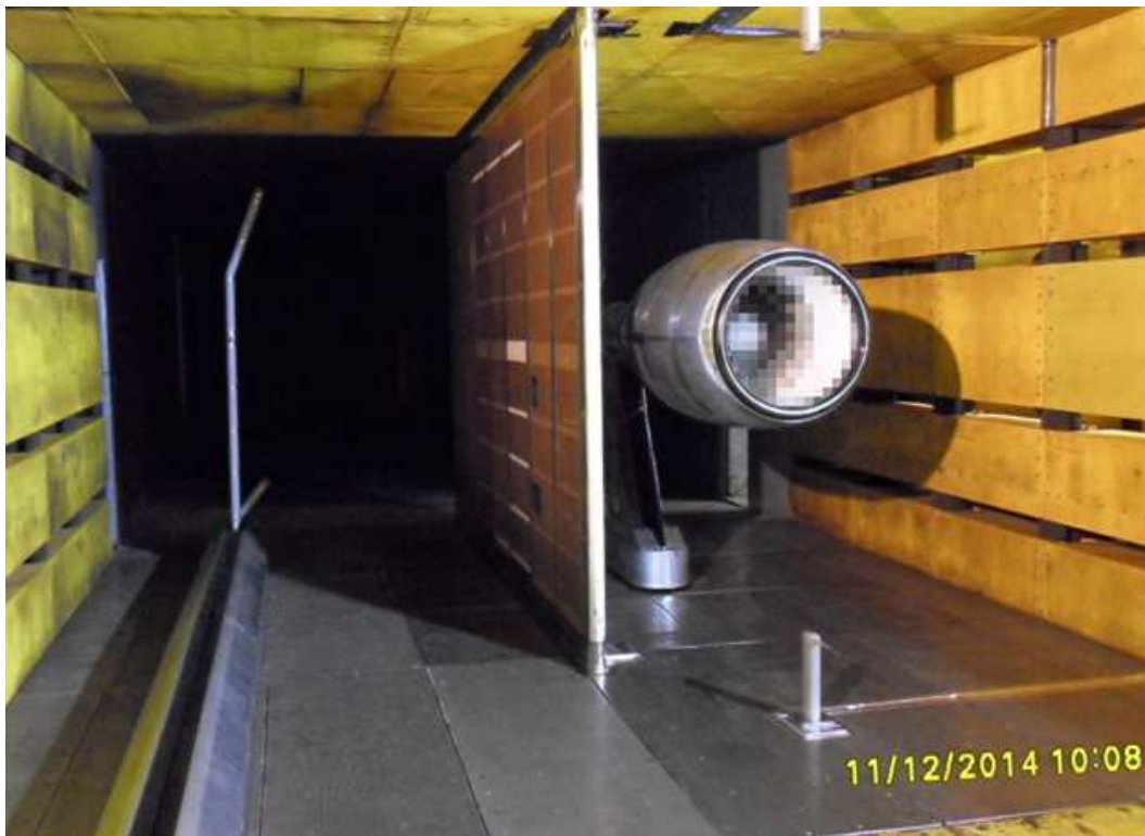
Figure 18: Barrier wall installed in the 9x15 LSWT.
