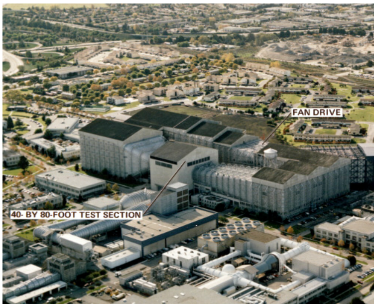
Figure 6. Overhead view of Arnold Engineering Development Complex NFAC.
